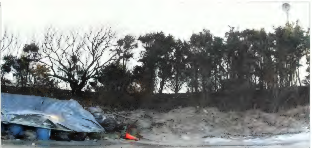
Figure 3.66. View looking south at engineered earthwork, NIKE launch site. South of the Warhead Building, a crescent-shaped earthwork rises to an elevation of twenty feet. The tips of the crescent wrap around the Warhead Building to the north and almost form a continuous landform with a northern earthwork (Olmsted Center, January 2009).
